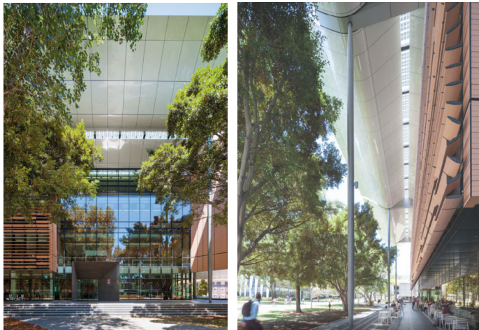
Figure 3-3-1 Tyree Energy Technologies Building (TETB)
