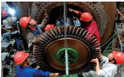
图为南京金陵石化对催化装置进行技术改造，更换新型烟机机组，新机组运行后可节电 2000 千瓦 / 小时 The picture shows Nanjing Jinling Petrochemical Company's technological transformation of a catalytic unit, the new smoke unit can save 2,000 kilowatts power per hour
